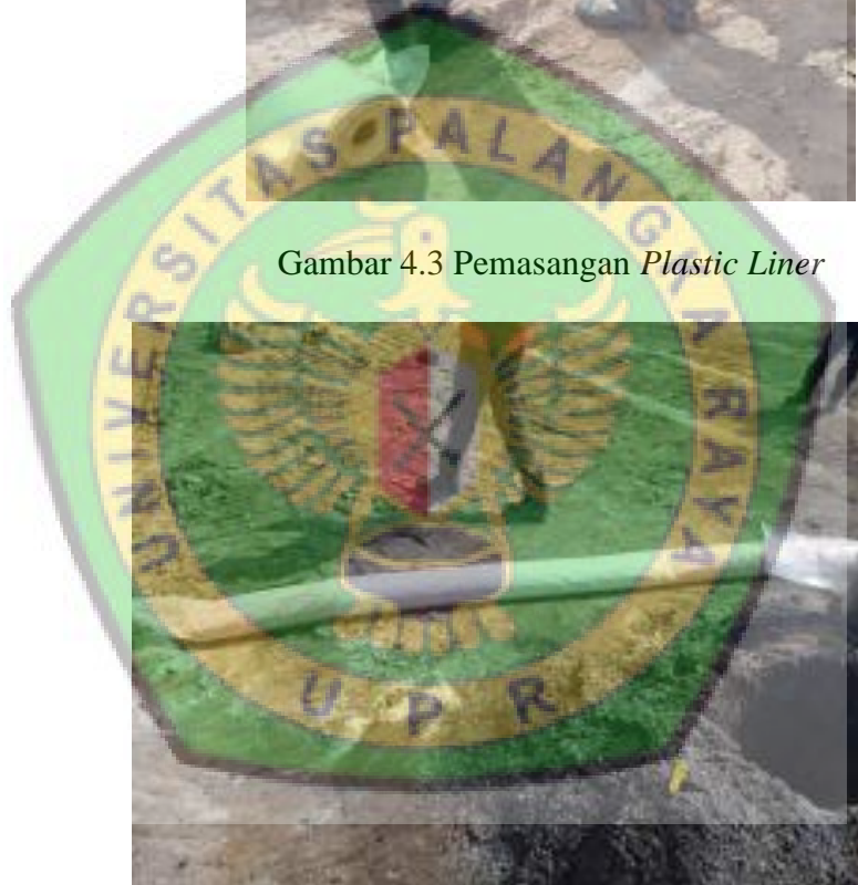
Gambar 4.4 Plastic Liner Berisi ANFO
